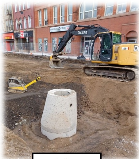
New Sanitary Maintenance Hole
